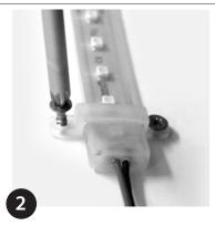
Place strip in clips and fix remaining screw. Do not over tighten.
