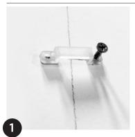
Mark and drill (if required) for screws. Fix clips with 1 suitable screw (min. 5 clips per metre or every 250mm/9.84").
