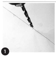
Mark and drill (if required) for screws (min. 5 clips per metre or every 250mm/9.84").
